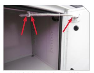
**B. Lubricate Spring Loaded Door Holders**
